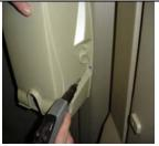
Fasten the 4 roll paperguard to panel using #17030 (3) Rivet, avdel black. Fasten papergaurd on the inside of the toilet. Using the top hole on the inside of paperguard and Transfer drill bottom two holes (one on each side) through paperguard and fasten to panel. Note: Be careful just to drill through first layer only.
